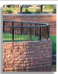
**Stone-Crete** walls mimic the look of natural stone with the versatility of concrete without the high cost of labor and materials. Its deep-relief texture and patented coloring process create an endless variety of designs and meet architectural specifications. Stone-Crete is also the formliner of choice for quality precast projects.
